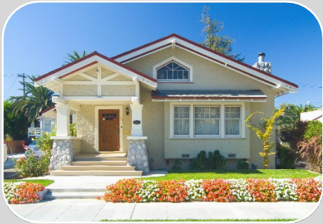
Stablized in place
