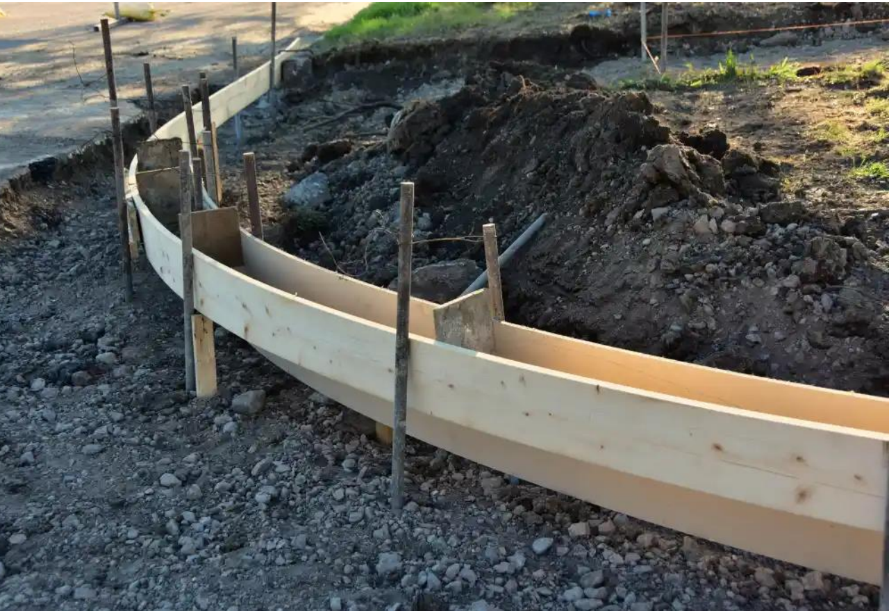
Curb and Gutter
