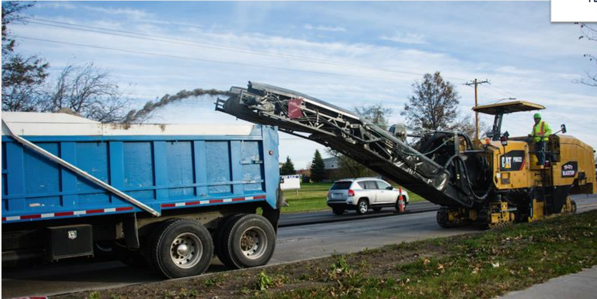
Asphalt Milling
